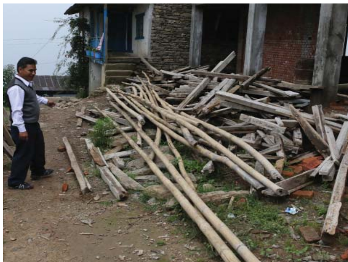
Photo (right): bamboo and salvaged wood used to build the frame for new TLCs at the Shree Durga School. The CGIS we supplied to the school was used for the roofing.
