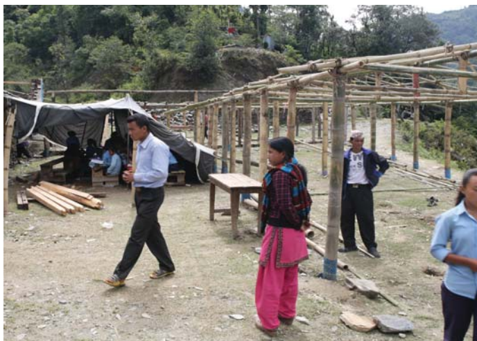
Photo (left two): top photos shows the blue CGIS loaded in the truck for transportation to the Shree Nabin School. Bottom photo shows the bamboo frame being prepared as TLCs.
