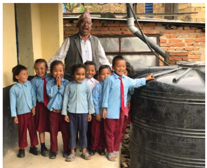
Photo (top): Installation of the 10,000 litre tanks at Bal Mandir. (opposite page top) Children and orphans from Bal Mandir during lunch break (bottom): LED projector being used to demonstrate laptops use skills to children in the new computer centre at Bal Mandir.
